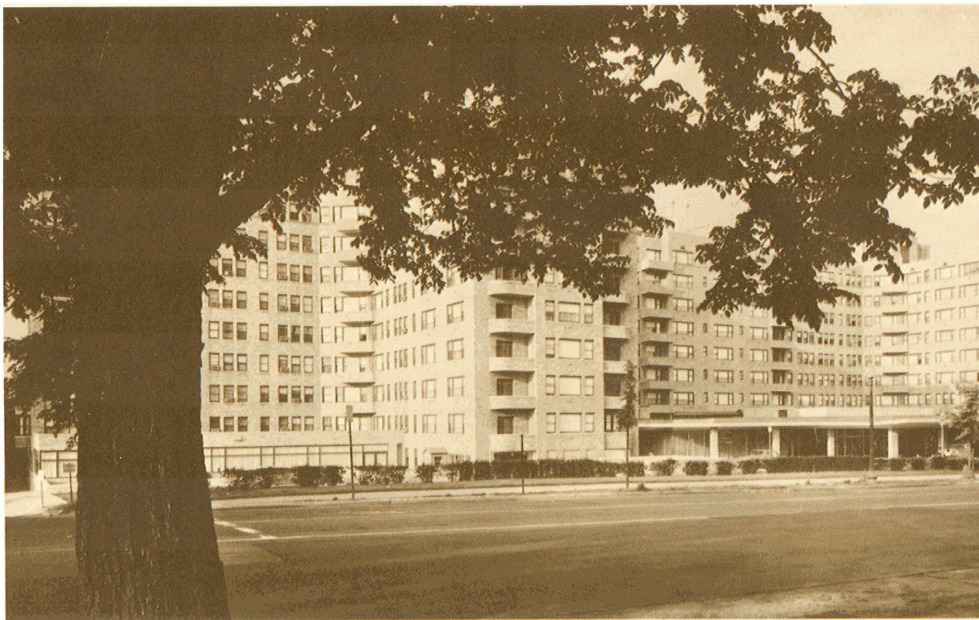
EXTERIOR VIEW OF THE SHOREHAM HOTEL, WASHINGTON, D. C., SCENE OF THE GRAND LODGE'S SESQUI-CENTENNIAL BANQUET, NOVEMBER 29, 1961, IN THE TERRACE ROOM. ON THIS OCCASION THE GRAND LODGE WAS HOST TO THE MASTERS AND WARDENS REPRESENTING ALL OF THE LODGES IN OUR GRAND JURISDICTION, AND THEIR LADIES.
